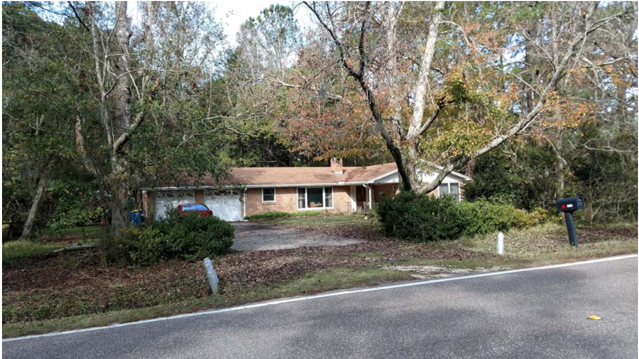
Single-family residential across Dunn Creek Road to the west
